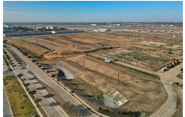
The future site of Port San Antonio's vertiport is seen in January. Credit: Port San Antonio
